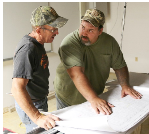
Paul McCullough, left, of Sandy Lake, a supervisor with general contractor Fred L. Burns, Shipperville, discusses blueprints with Steve Hawk, of Clarion, and also of Fred L. Burns, inside BC3 @ Cranberry in Cranberry Township on Tuesday, July 17, 2018.
