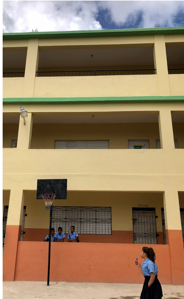
Students are shown in February 2020 outside the three-story school built in 2008 by Dr. William DiCuccio’s mission in Villa Hermosa, Dominican Republic. The school educates 400 children each year in kindergarten through sixth grade. DiCuccio, a Butler County Community College trustee from Gibsonia, has been named one of six 2020 Alumni of Distinction by Saint Vincent College, Latrobe, where he earned a bachelor’s degree.
